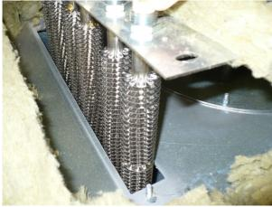
9.Replace Heater- If bad – check heater for continuity with wires removed
